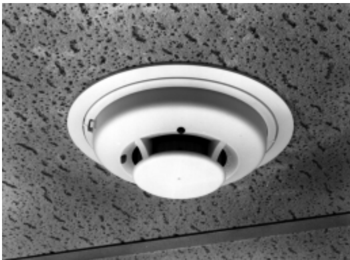
Figure 3. Adapter bracket covers previous detector footprints and flawed installations.
