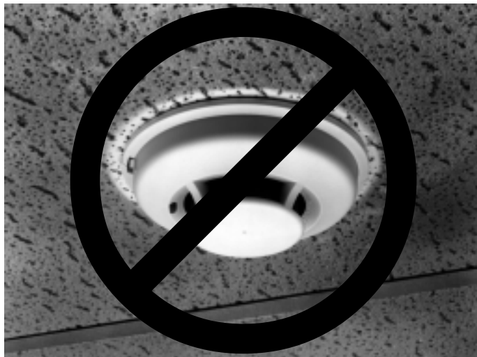
Figure 4. Detector without adapter bracket
