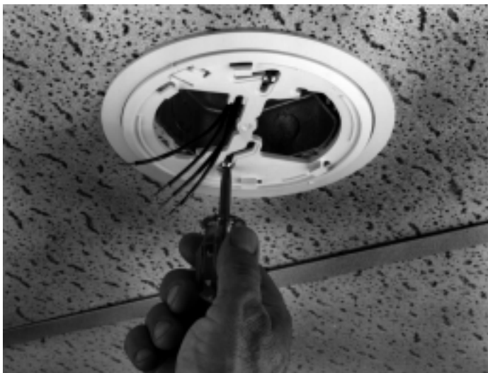
Figure 1. Install adapter bracket between ceiling and mounting bracket.
