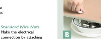
Wide-based wing nuts secure the speaker assembly to the ceiling tile.
