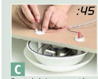
Two standard wire nuts connect the speaker wires to the mounting studs, making the electrical connection. That's all it takes!
